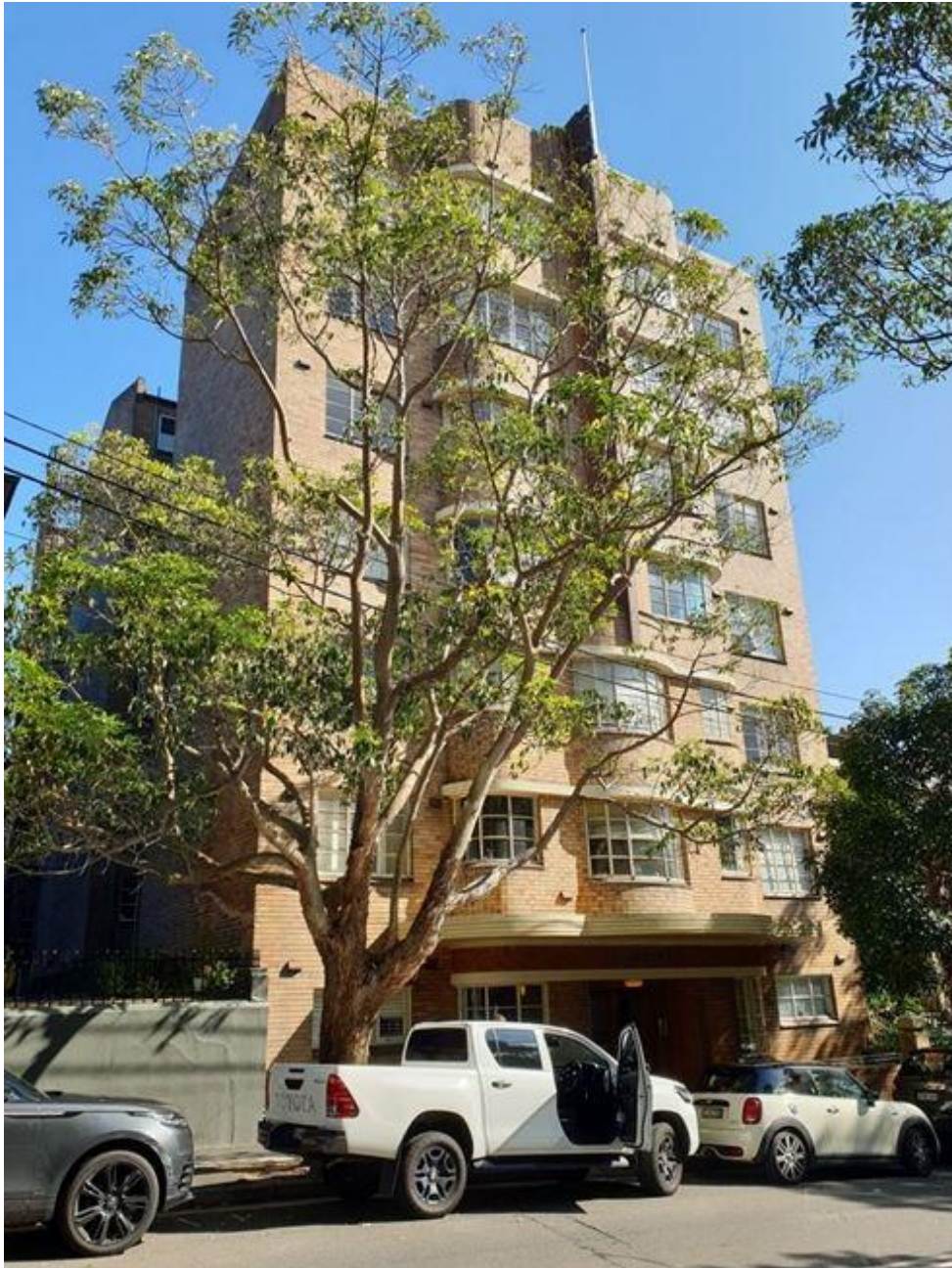
Figure 3: The adjoining residential flat building at 349 Liverpool Street (local heritage item), viewed from the northern side of Liverpool Street, facing south-west
