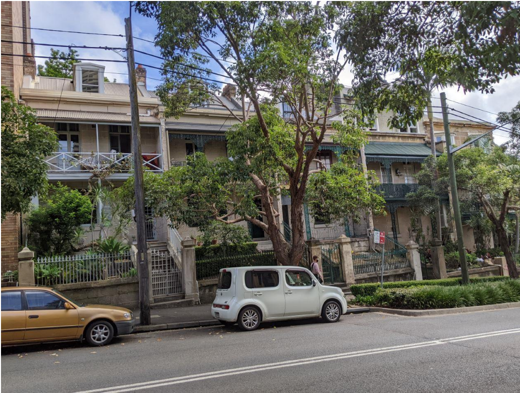
Figure 6: The residential flat building and terraces at 337-339, 341, 343, 345 Liverpool Street (all local heritage items, from right to left), viewed from the northern side of Liverpool Street, facing south-west
