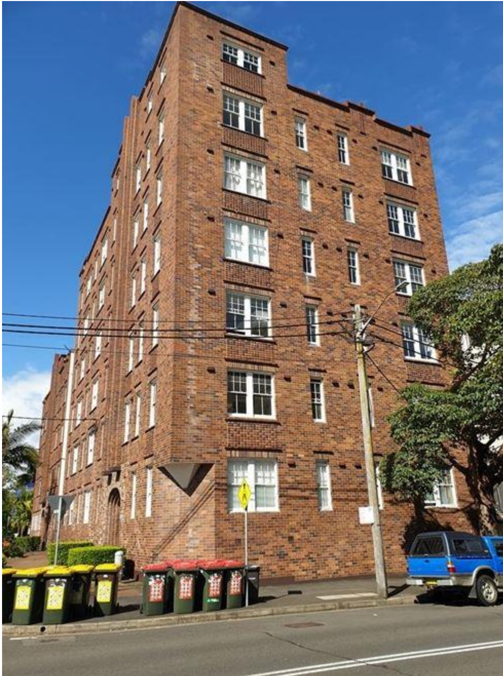
Figure 5: The residential flat building at 5 Darley Street (local heritage item), viewed from the northern side of Liverpool Street, facing south-west
