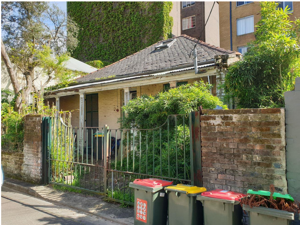
Figure 14: The adjoining cottage at 1 Darley Place (local heritage item), viewed from the southern side of Darley Place, facing north-west
