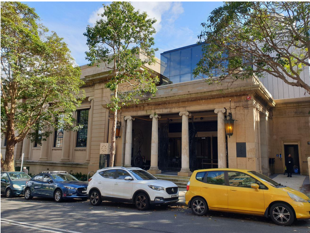
Figure 7: The office premises at 262 Liverpool Street (local heritage item), viewed from the southern side of Liverpool Street, facing north-west
